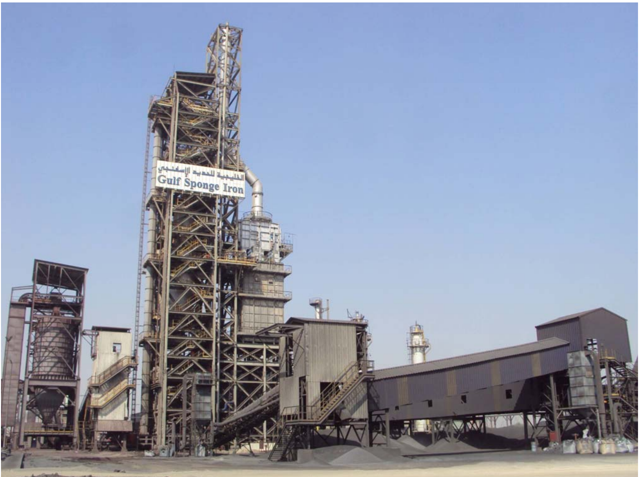
Gulf Sponge Iron Micro-Module DRI Plant at Mussafah, Abu Dhabi, UAE
