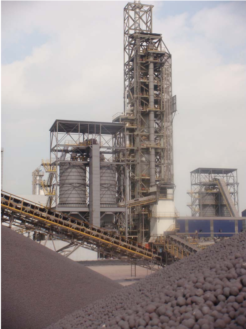
Gulf Sponge Iron Micro-Module DRI Plant at Mussafah, Abu Dhabi, UAE
