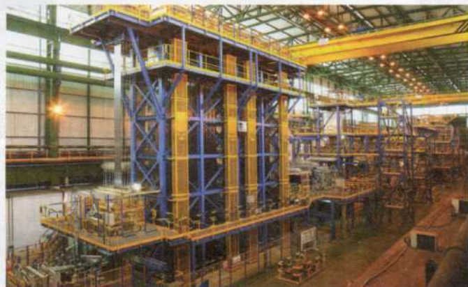
4 Double loop accumulator tower at Aceralia
