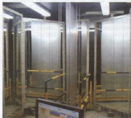
5 Vertical Inspection Station
